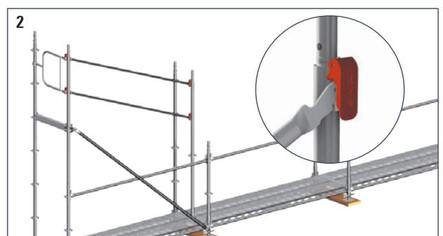
Insert the guardrails into the already fitted AGS standard. Despite the bar being closed, the guardrail can be assembled from the secured level. The guardrails are then connected to the next AGS standard.
